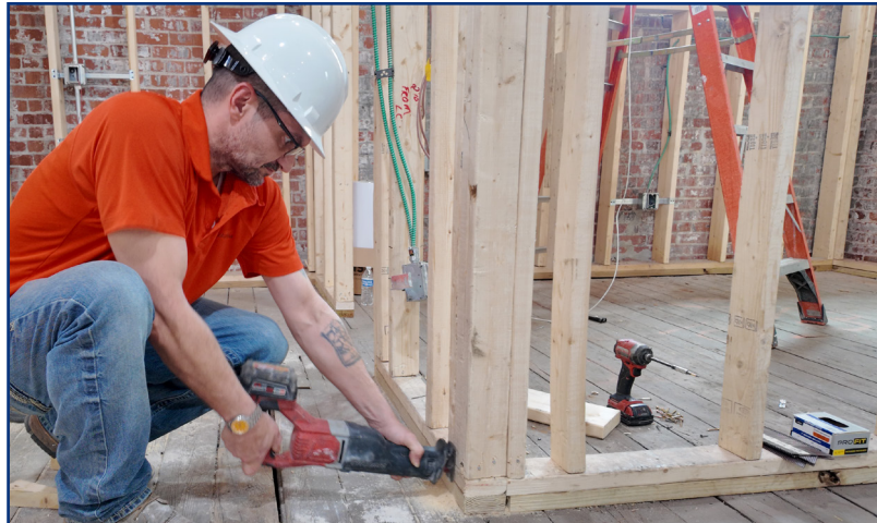
Robert Perkins with Patterson Horth Inc. works on framing at Indiana Health Centers in downtown Seymour as part of a $3.443 million Lilly Endowment Inc. GIFT VIII Implementation Grant project.
